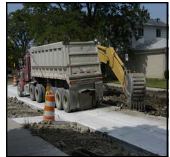
Construction activities during the past fiscal year.
